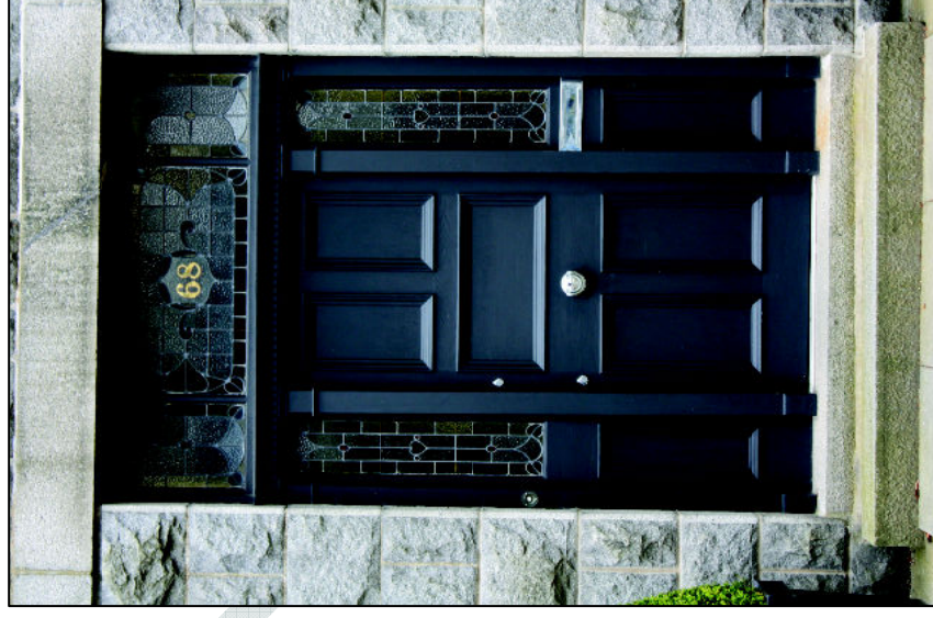
Historic glass should be reused where this contributes to the character of a building
